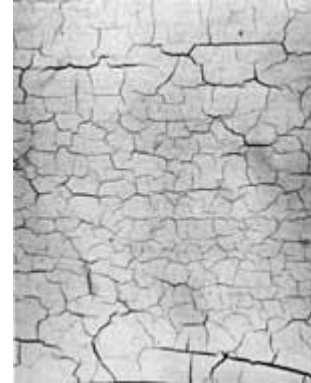
Crazing--or surface cracking--is an exterior surface condition which can be successfully treated by sanding and painting. Photo: Courtesy, National Decorating Products Association.
